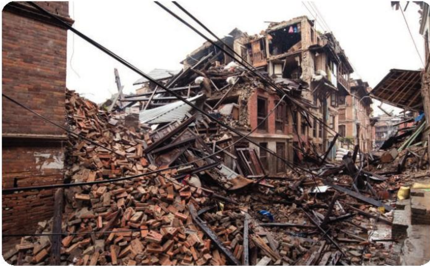
◀ This photograph was taken after the 2015 earthquake in Nepal, which had a magnitude of 8.1
